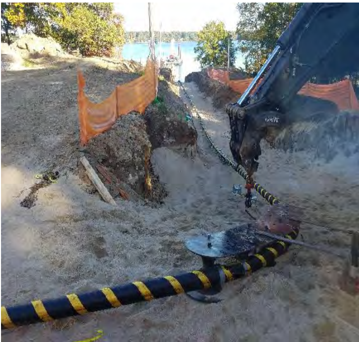
Fig 19: Cable pull on the west side of the Bay. Viewing east. (10-15-19).
