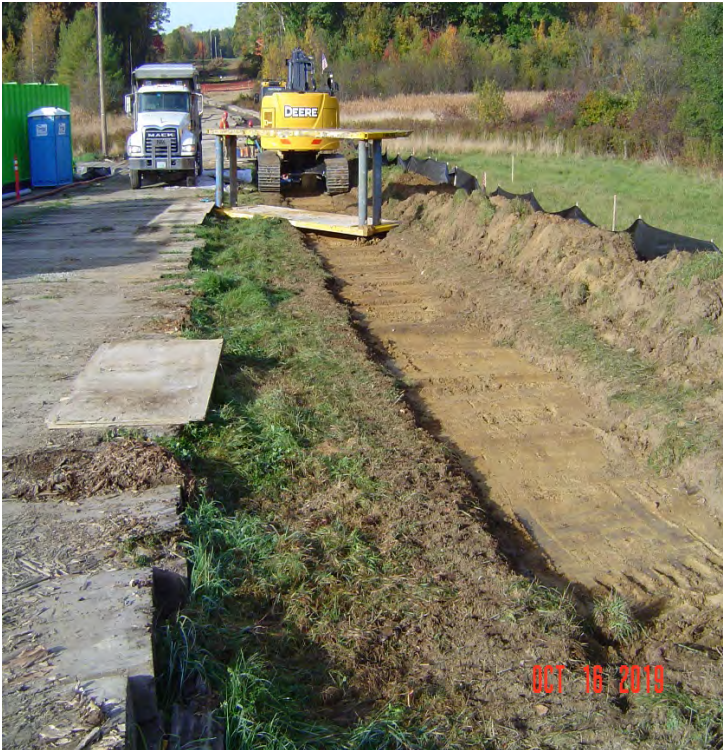
Fig 23: Stripping topsoil in agricultural zone at Frink farm. Viewing west. (10-16-19).
