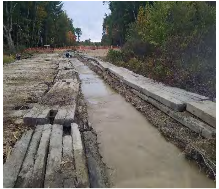
Fig 2: Float fill in trench at Str. 106. Viewing east. (10-11-19).
