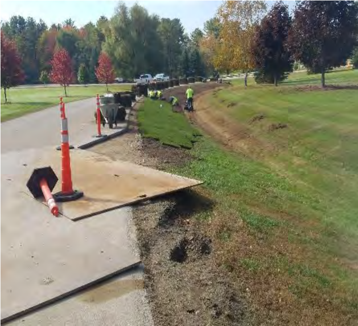
Fig 13: Crew placing sod over restored trench along Gundalow landing. Viewing west. (10-14-19).
