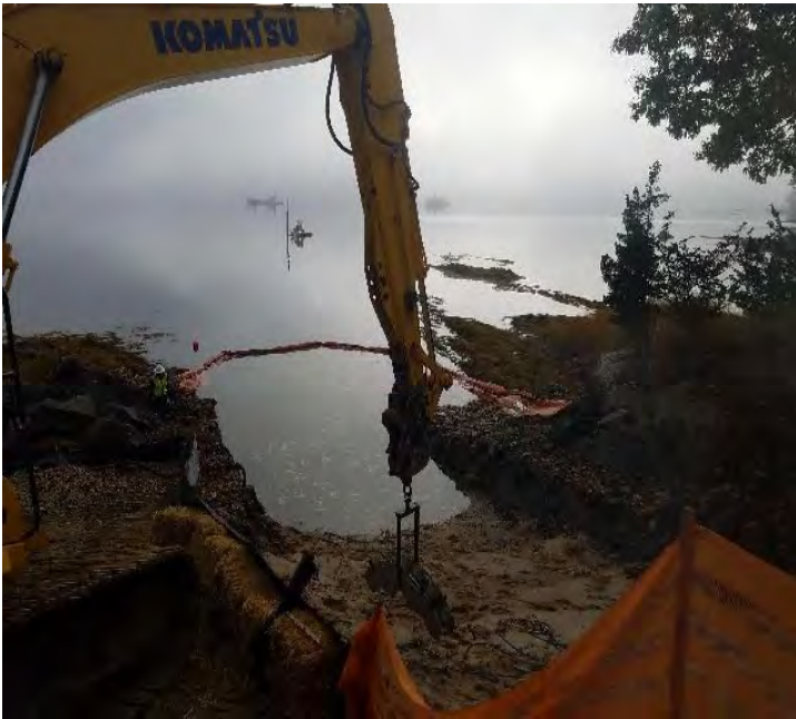
Fig 9: Prepping to pull the cable at the Getchell property. Viewing east. (10-14-19).
