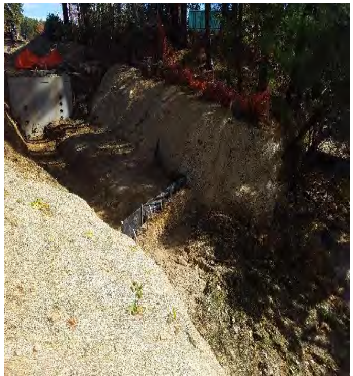
Fig 32: Sediment controls in trench on the east side of the Bay. Viewing east. (10-18-19).
