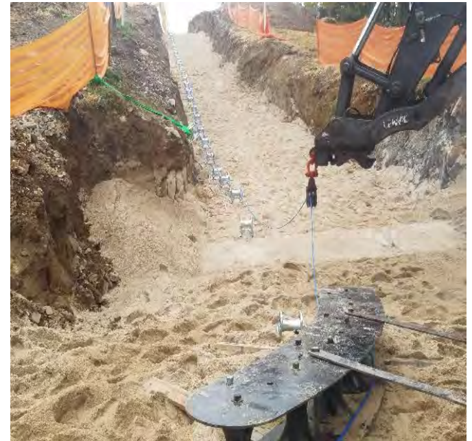
Fig 8: Prepping to pull the cable at the Getchell property. Viewing east. (10-14-19).
