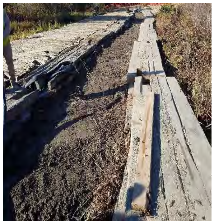
Fig 16: Restoring wetland NW 16. Viewing west. (10-15-19).
