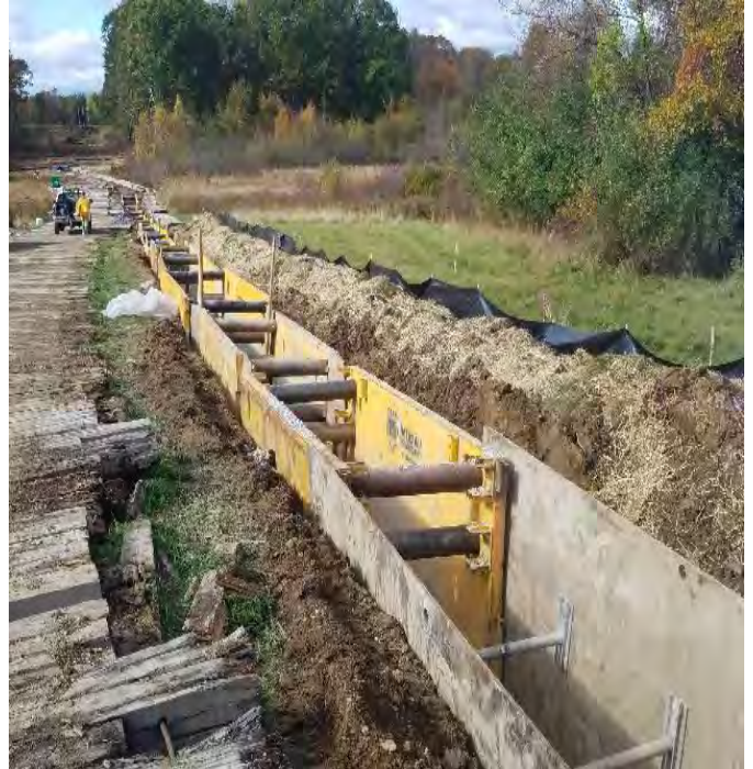
Fig 30: Trenching activities in upland agricultural zone at Frink farm. Viewing west. (10-18-19).
