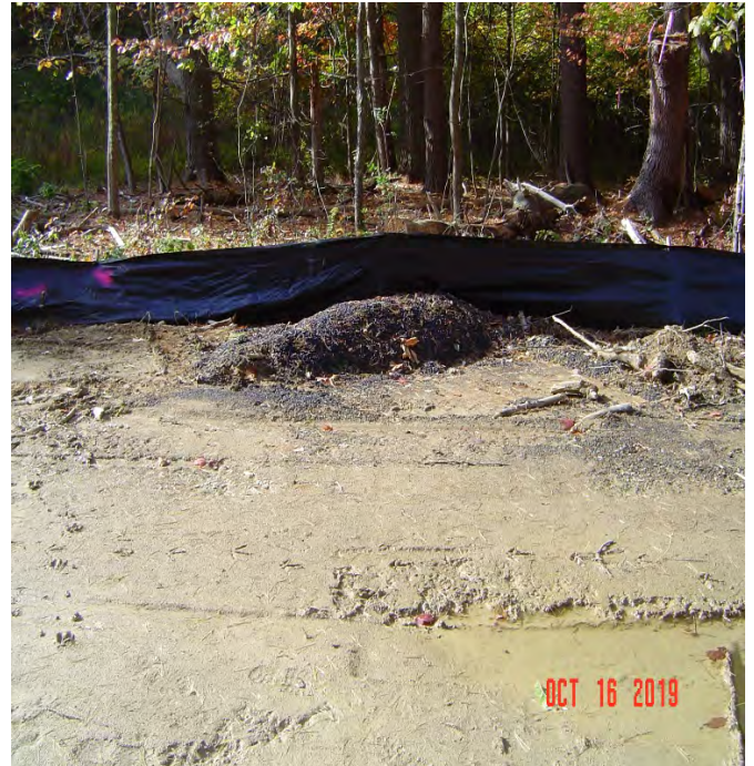
Fig 26: Cold patch asphalt needs to be removed at Flynn Pit. Viewing south. (10-16-19).
