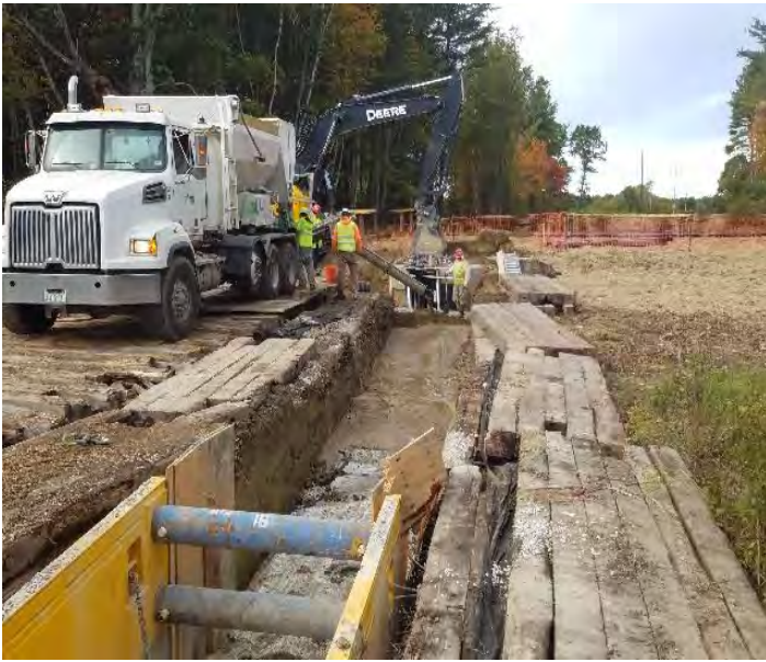
Fig 1: Pouring float fill in trench at Str. 106. Viewing west. (10-11-19).
