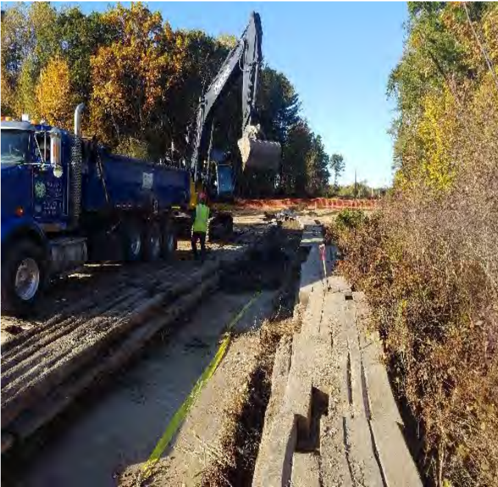
Fig 15: Restoring wetland NW16. Viewing west. (10-15-19).
