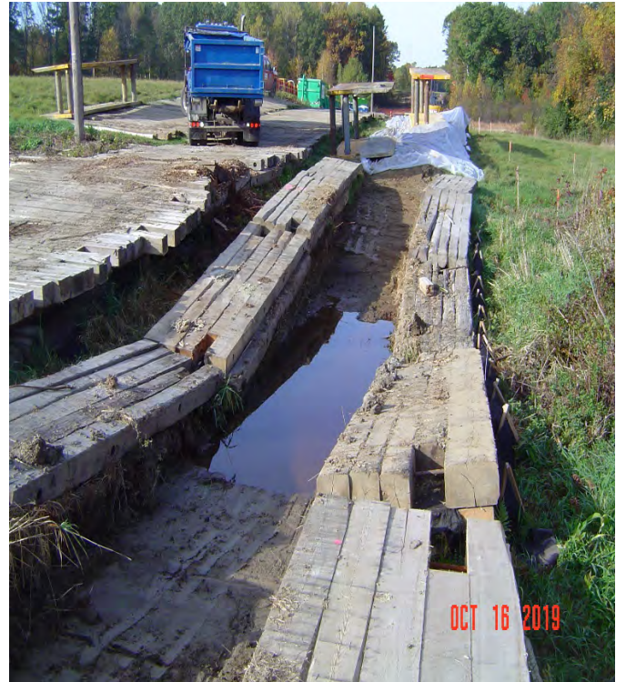
Fig 24: Stripping topsoil through wetland NW 18. Viewing west. (10-16-19).
