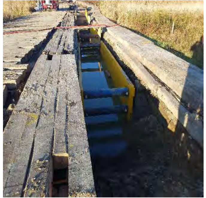
Fig 14: Accumulation of groundwater in trench at Frink farm. Viewing west. (10-15-19).
