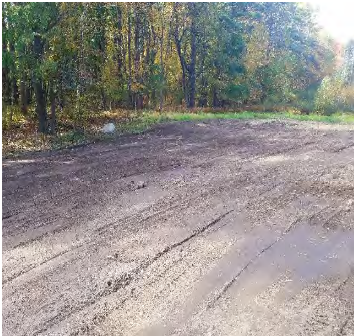
Fig 11: Spreading loam at Str. 100. Viewing west. (10-14-19).
