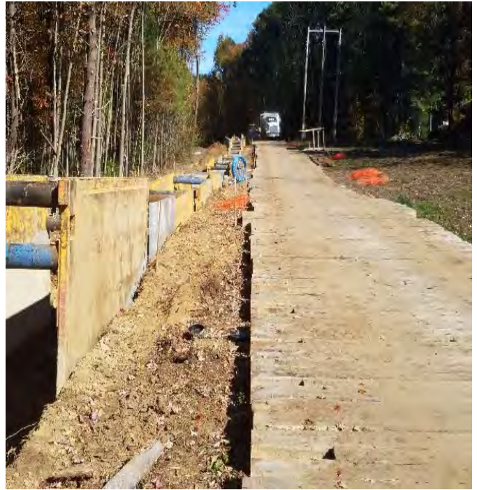
18: Trenching activities from Str. 107 westward. Viewing east. (10-15-19).
