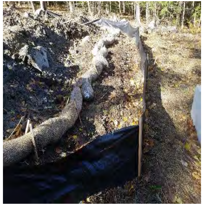
Fig 28: Sediment controls downslope from Str. 29. Viewing west. (10-18-19).
