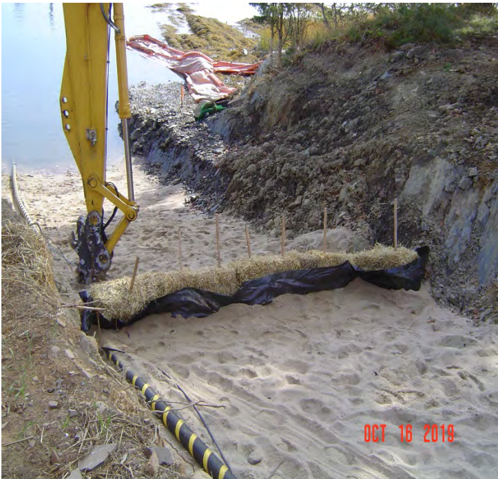
Fig 27: Sediment controls on the west side of the Bay. Viewing east. (10-16-19).
