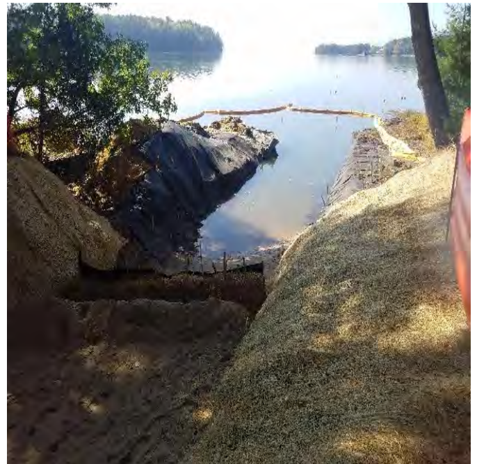
Fig 12: Sediment controls on the east side of the Bay. Viewing west. (10-14-19).
